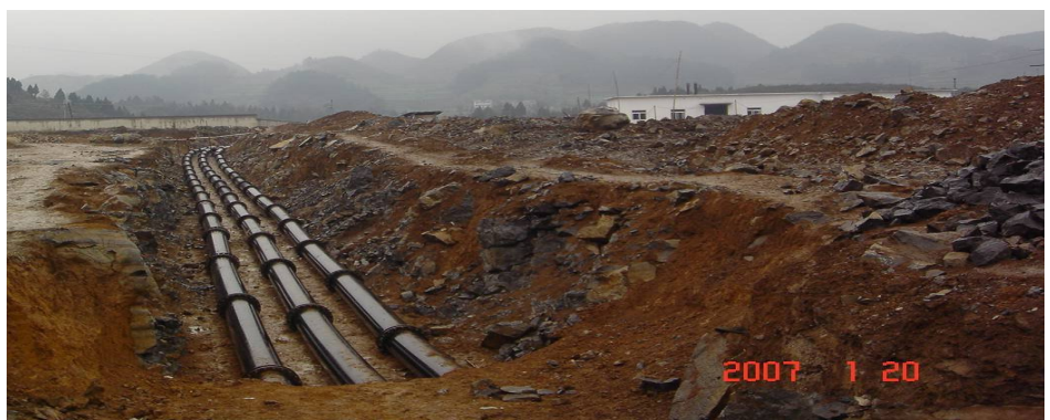
Pipes paved for coal mine methane drainage in Guizhou. Province.
