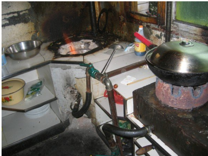
Figure 5: CMM used in kitchen at Coal Mine C
