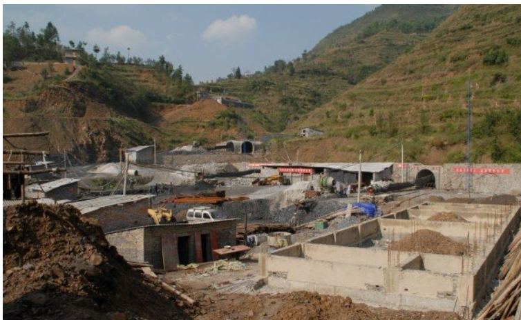
Figure 3: Coal Mine B under construction
