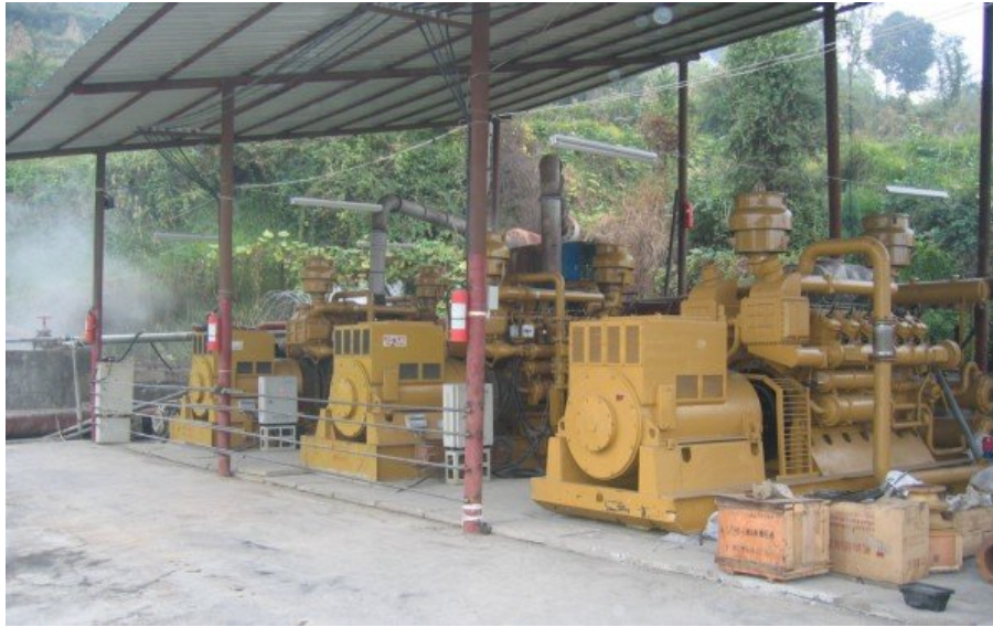
Figure 4: CMM Gas engines at Coal Mine C
