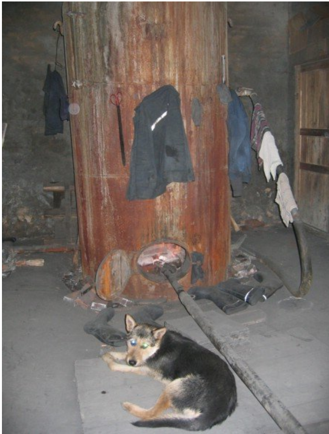
Figure 6: CMM also used for boiler at Mine C
